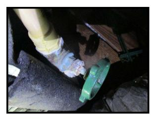
The T&P valve drain line was connected in to the PVC pan drain line.
