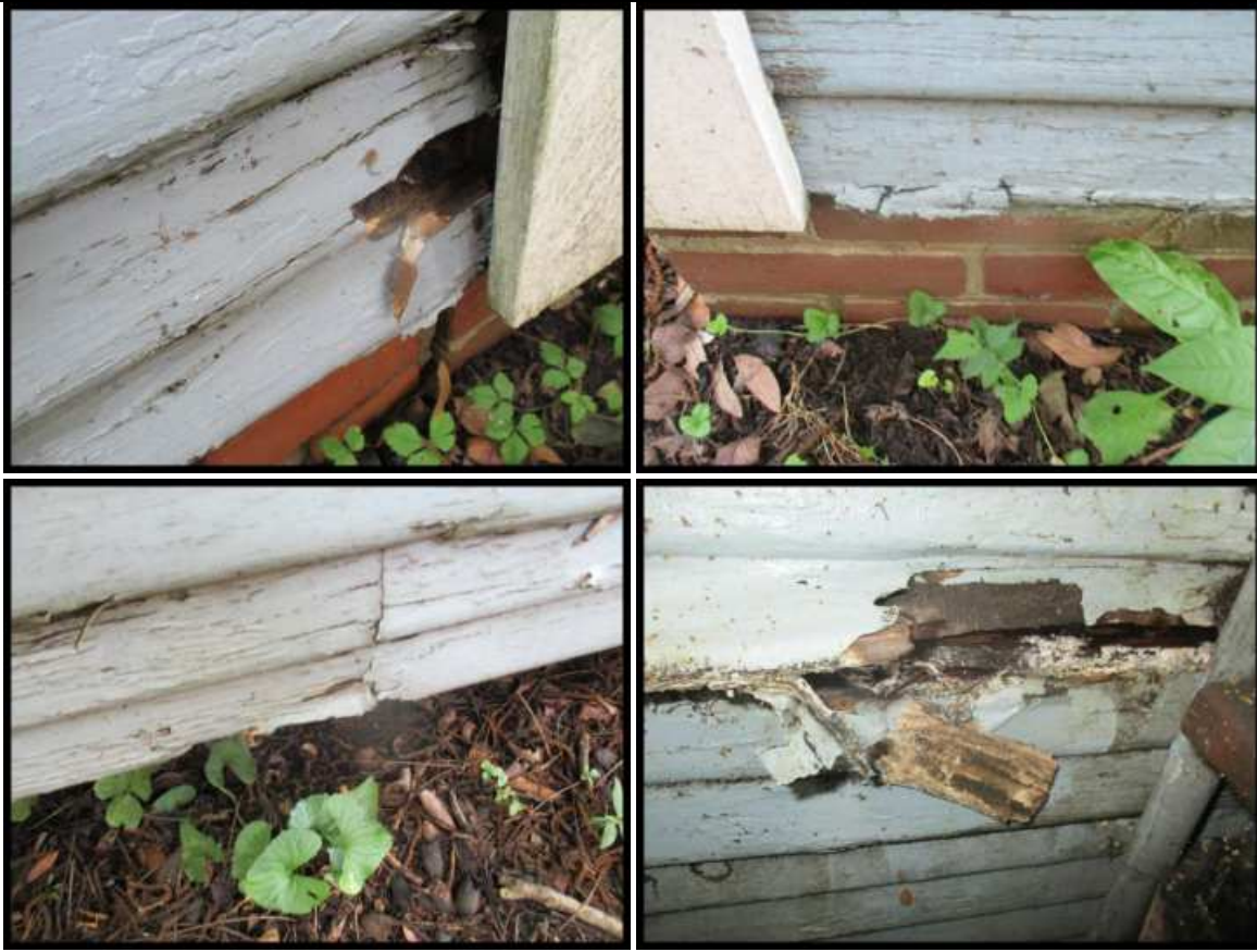
TRIM AND SOFFIT CONDITION Damage was noted in areas of the trim and soffits. Examples pictured.
