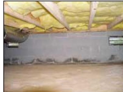
Much better than the typical crawl space encountered in the field, the wall-vented control houses in this study had well-installed insulation, 100 percent ground vapor retarder coverage of the soil and no problems with intrusion of liquid water from the outside.
